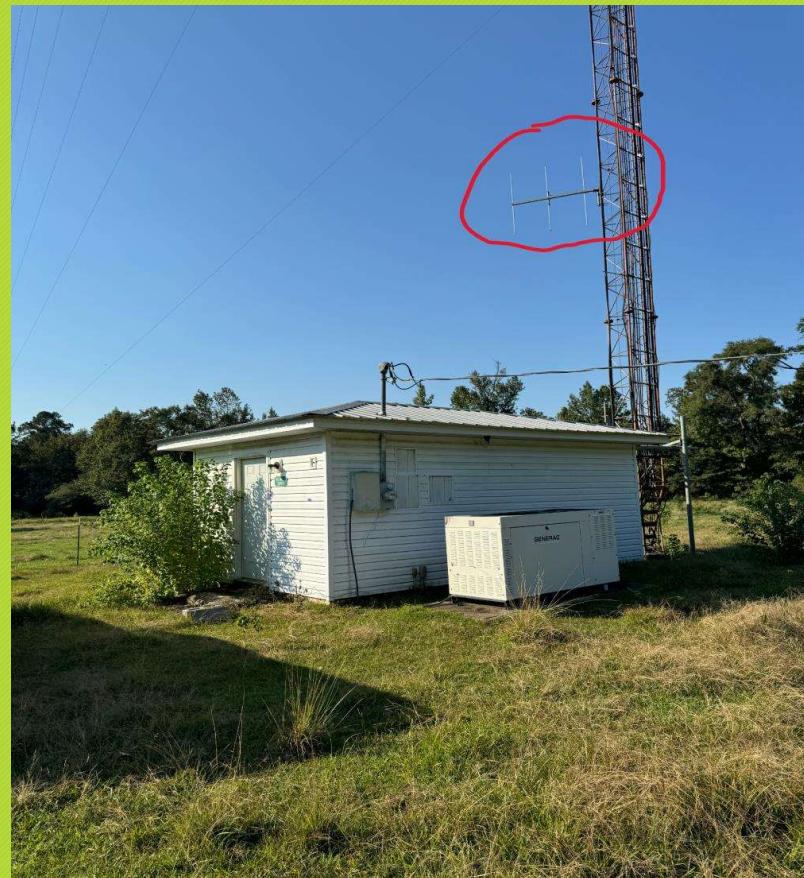
Rabun Shack & Tower showing UHF Yagi
